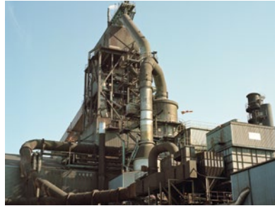
2. Mineral weighing—blast furnace
